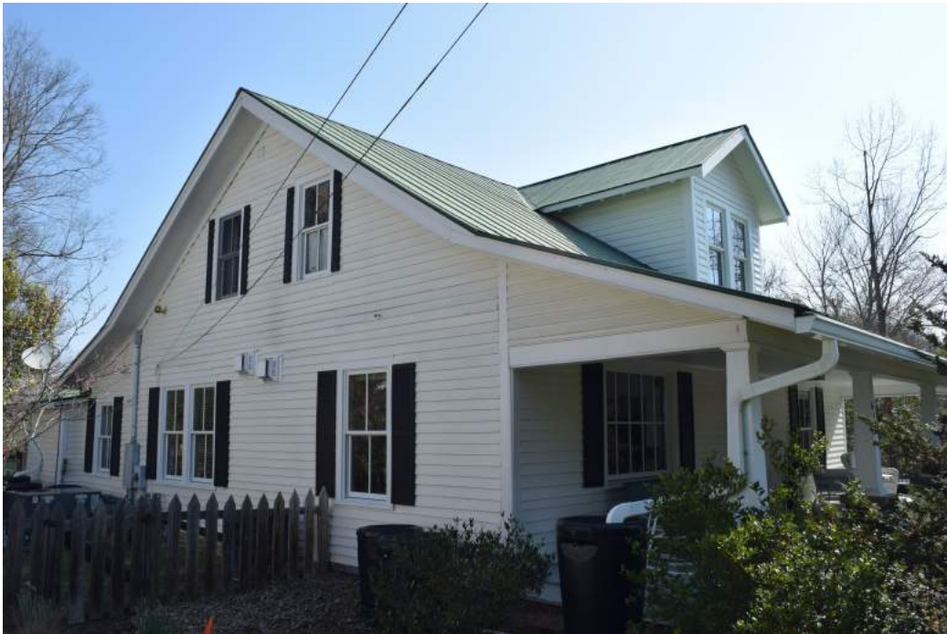
Figure 12: West corner of front of house, view to the east
