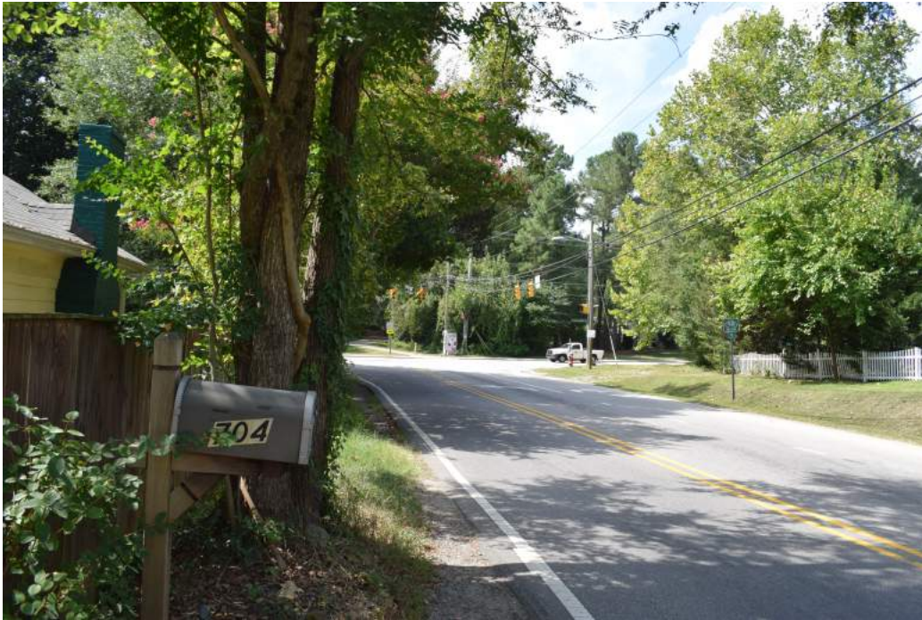
Figure 7: Estes Drive Extension with view towards North Greensboro Street, view to the southwest
