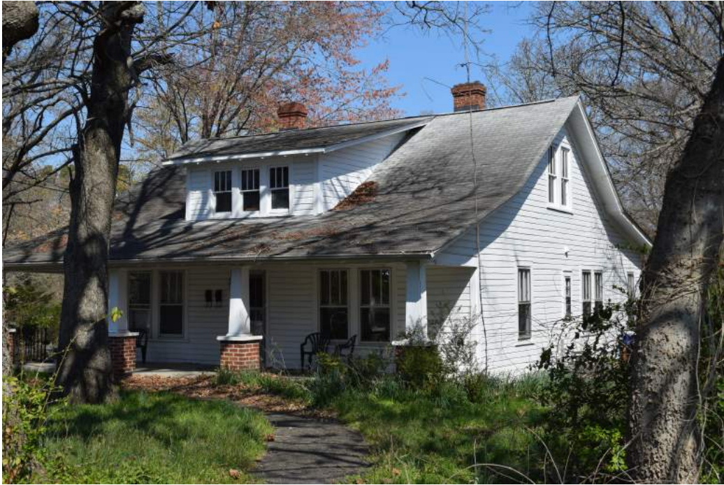
Figure 9: Bungalow at 401 Poplar Avenue, view to the north
