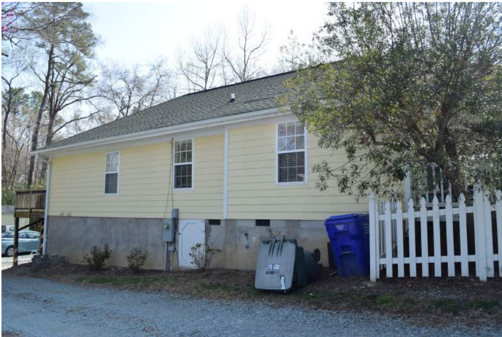
Figure 29: West elevation, view to the east
