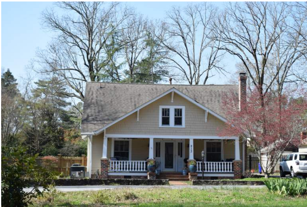
Figure 8: Bungalow at 213 Hillsborough Road, view to the southwest
