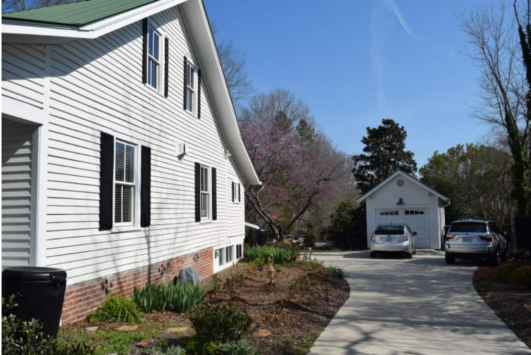
Figure 19: South elevation of house, driveway, and modern garage, view to the northeast
