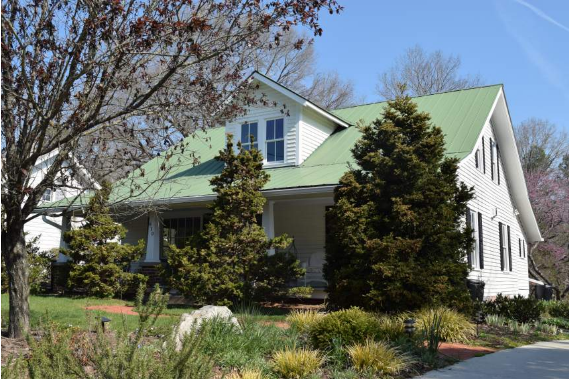
Figure 7: South (front) elevation of the Braxton House, view to north
