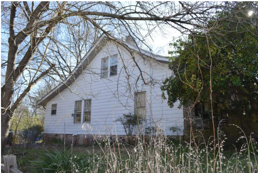
Figure 24: West elevation, view to the northeast
