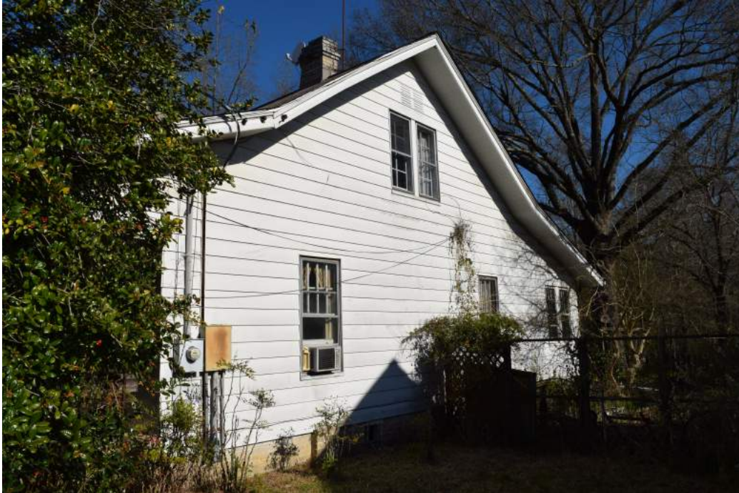
Figure 25: East elevation, view to the northwest
